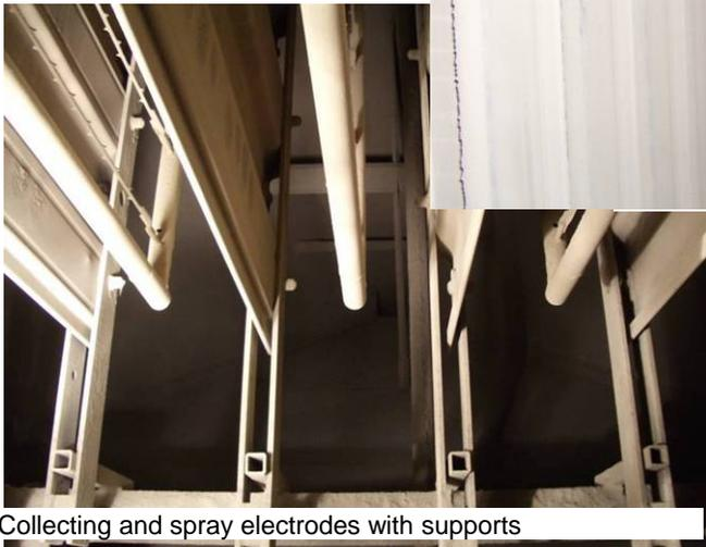
Collecting and spray electrodes with supports
