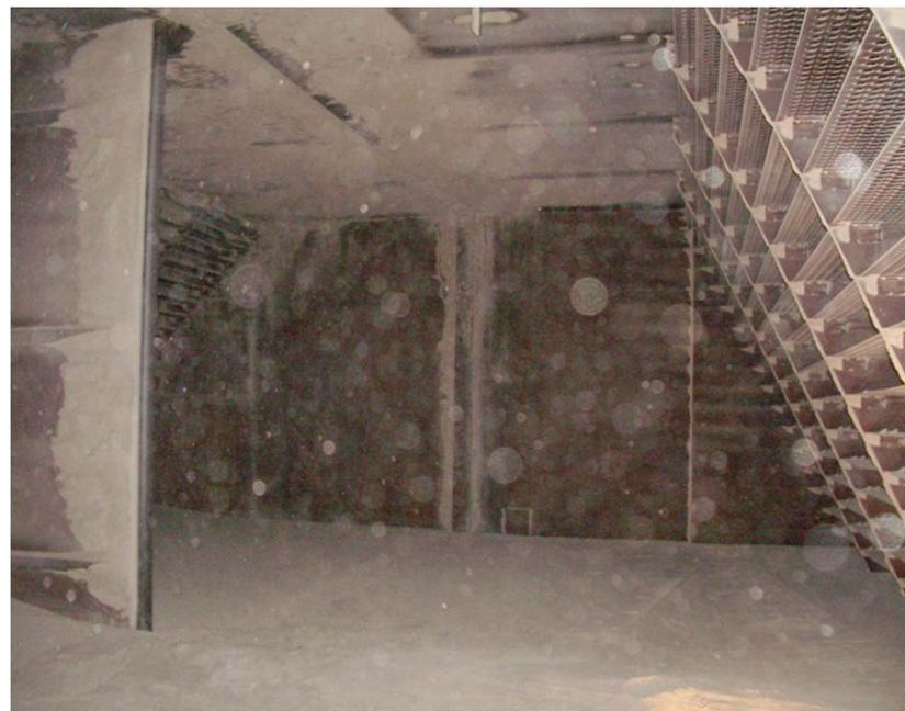
Perforated guide vanes and dividing wall for distribution to two ESP trains
