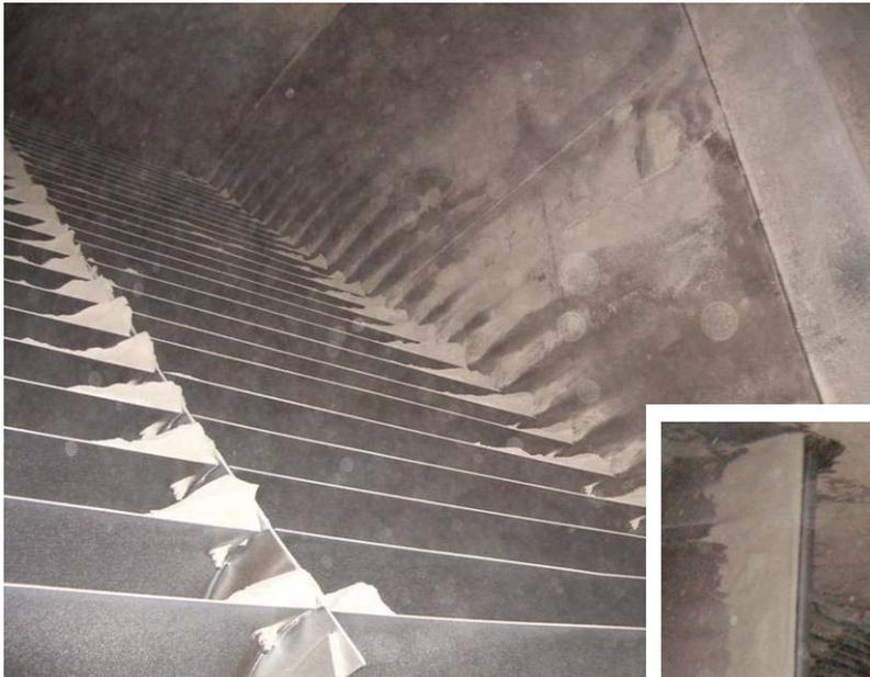
Guide vane level in duct section between air heater and ESP
